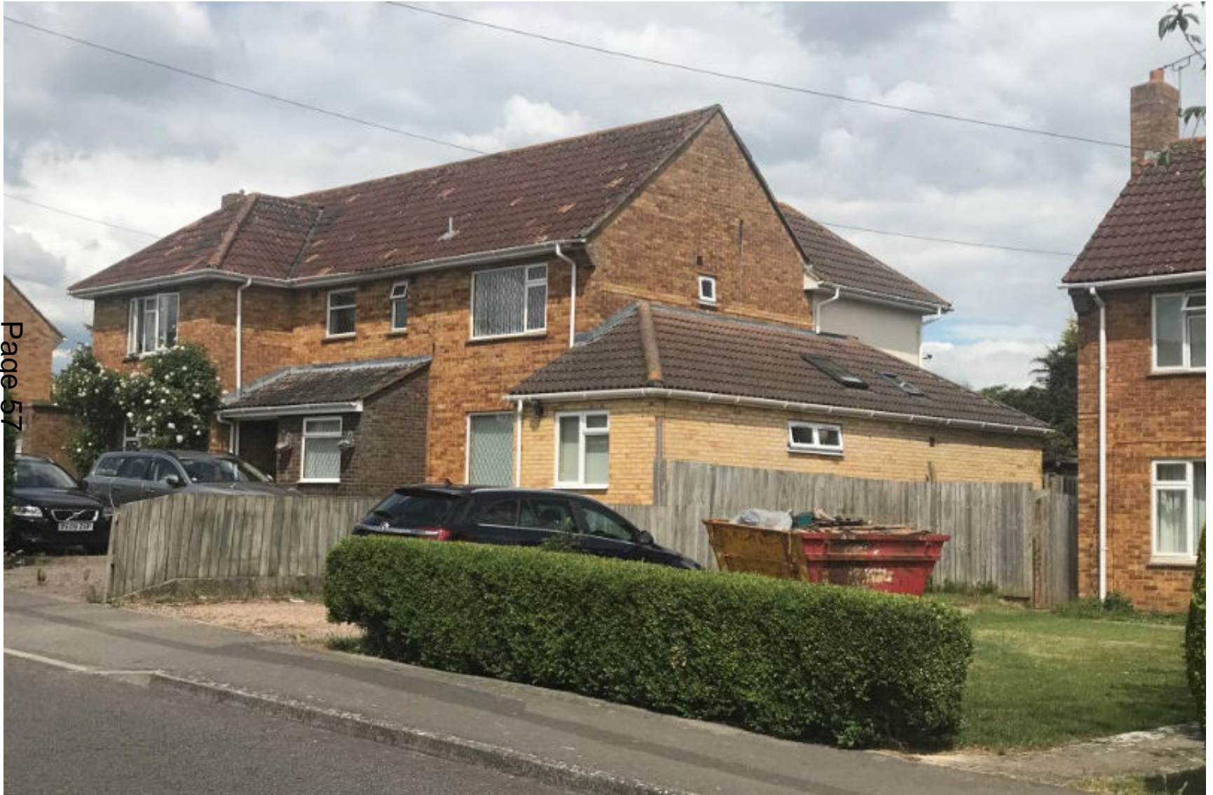
Photo showing existing single and two storey extensions within the existing street scene
