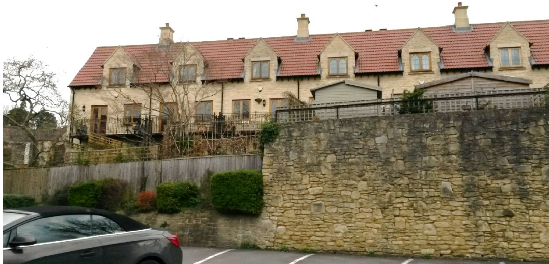
Rear of 1-6 Mill Lane
