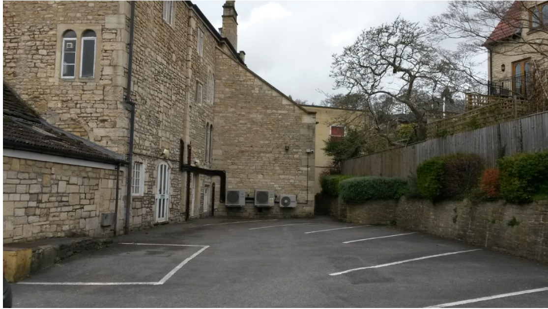
Rear of Manvers House from car park
