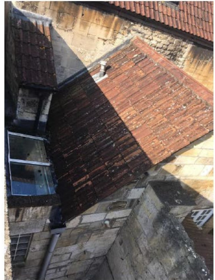
North Wing, Manvers House. Skylight to No. 1-2 Kingston Rd.
